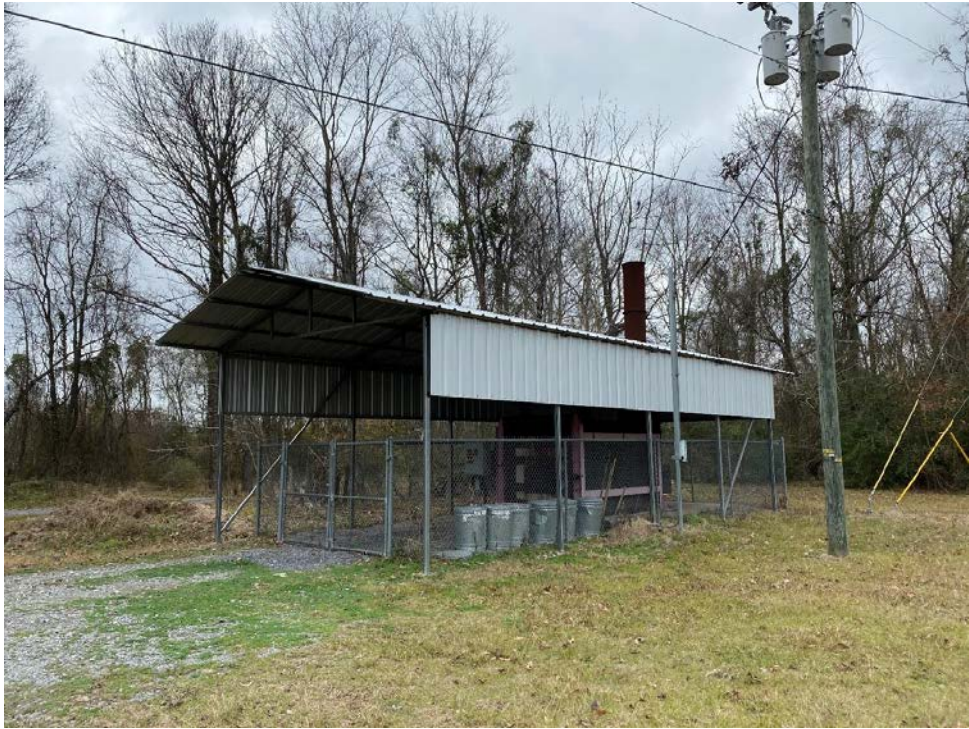
The LSP training center consisting of a slab with an incinerator.
