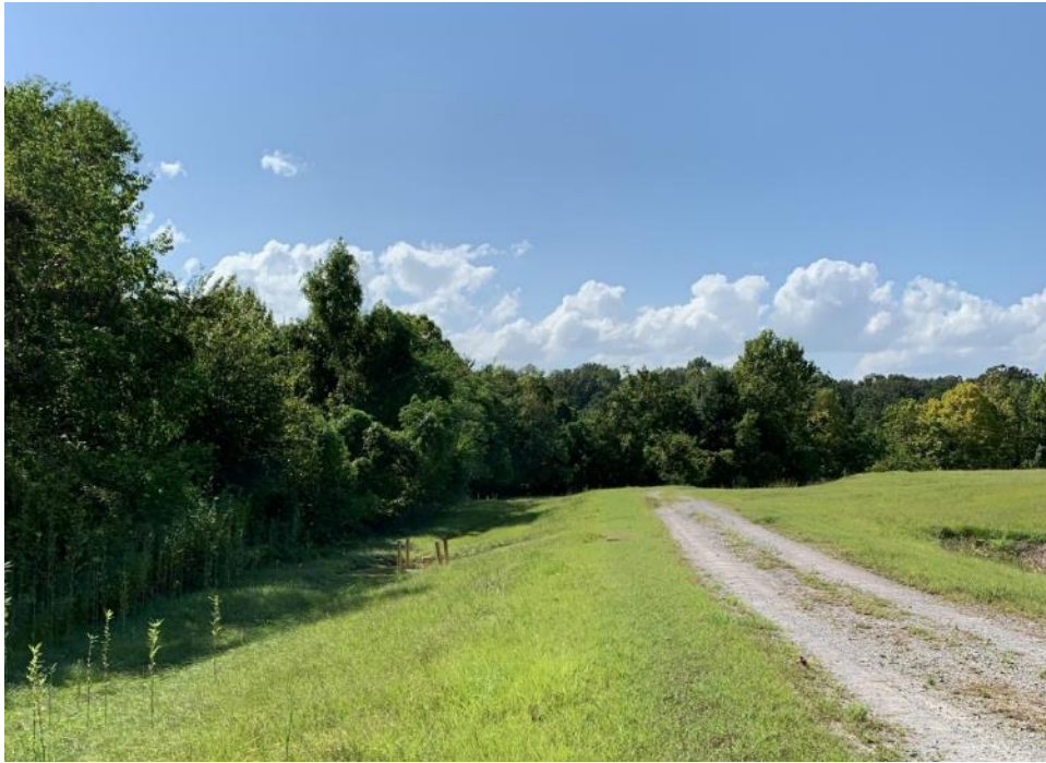
Capped borrow pit at the Scenic OU
