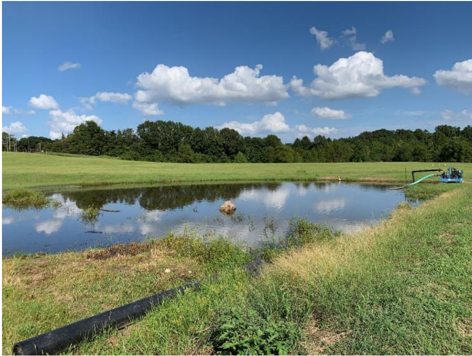
Stormwater catchment basin at the Brooklawn OU that is pumped and treated
