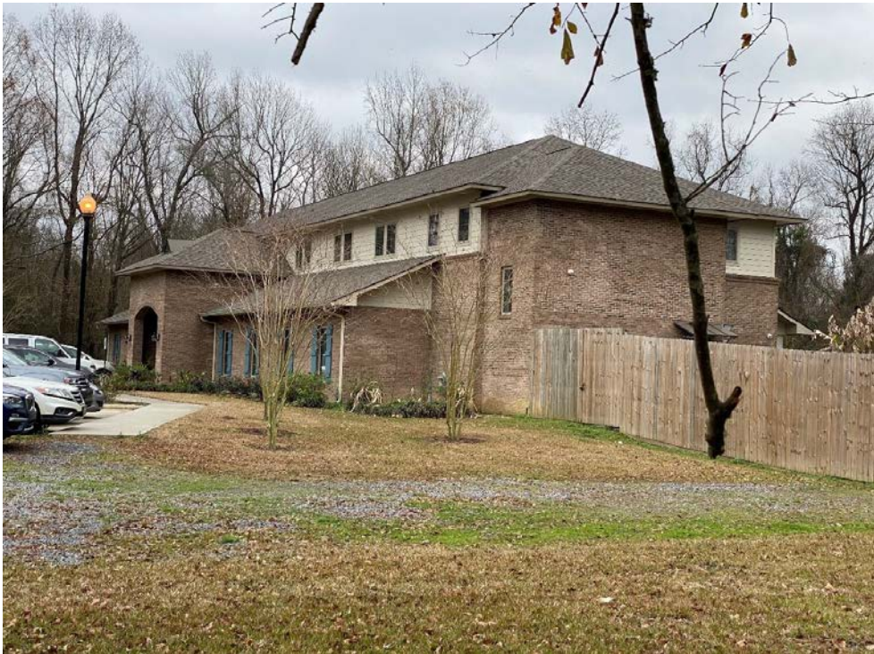
Occupied building east of the DTZ
