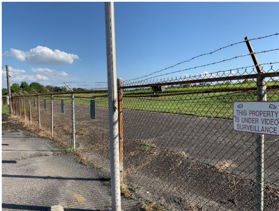
Fencing along the northern edge of the capped area at the Brooklawn OU
