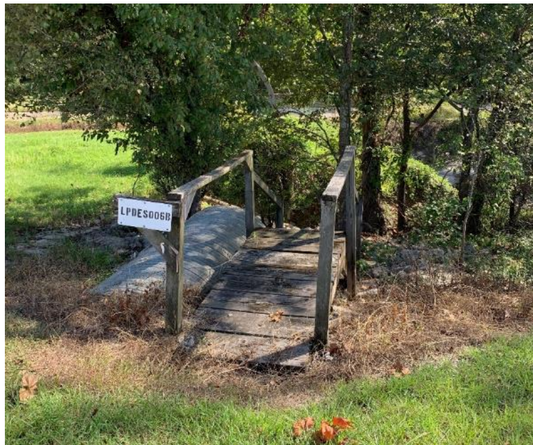
LPDES Outfall 006B at the Brooklawn OU
