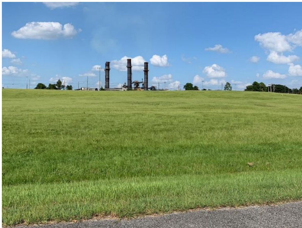
Filled upper lagoon at the Brooklawn OU, with recovery well field in the background
