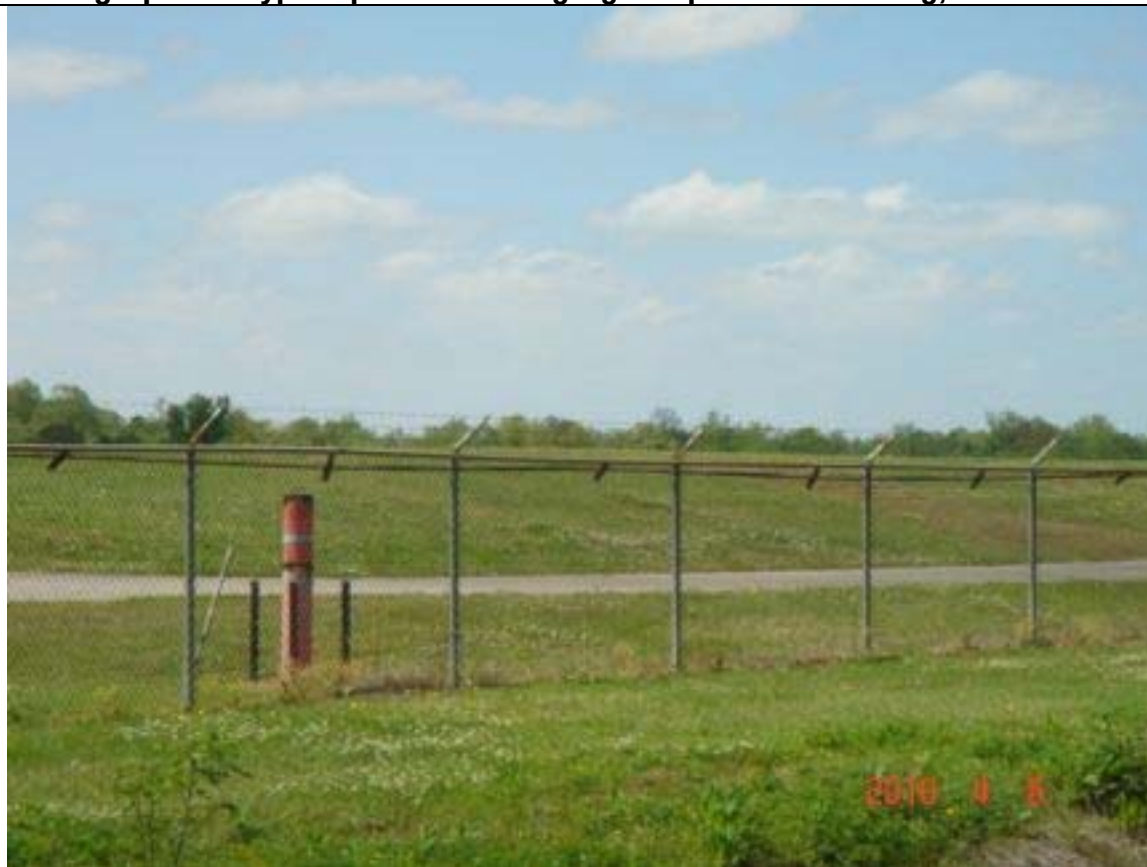
Photograph 4 – North Perimeter Fence, Brooklawn OU, South 4/6/10
