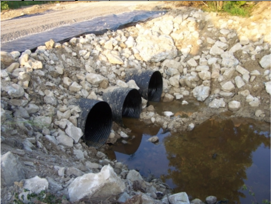
Photograph 28 – Bridge Construction, Scenic OU, Southwest 6/1/10
