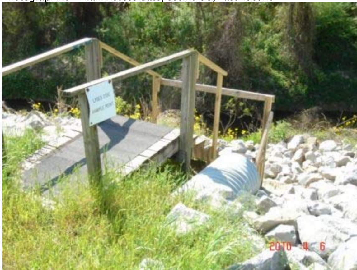
Photograph 20 – LPDES Outfall 013C, Scenic OU, East 4/6/10
