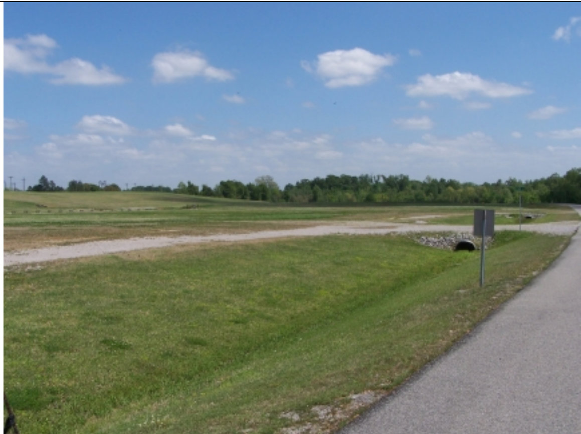
Photograph 9 – South Levee Road, Brooklawn OU, East 4/6/10
