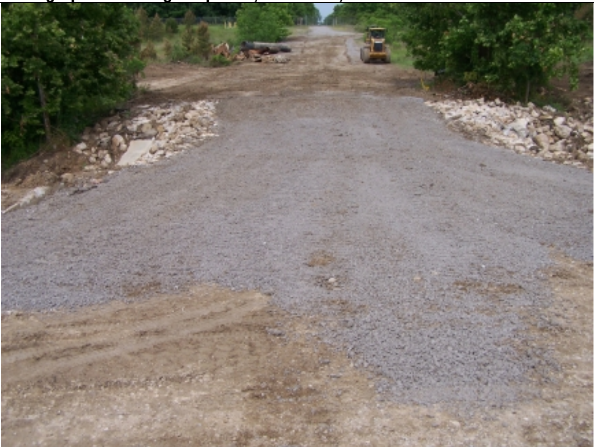
Photograph 30 – Bridge Repaired, Scenic OU, West 6/3/10
