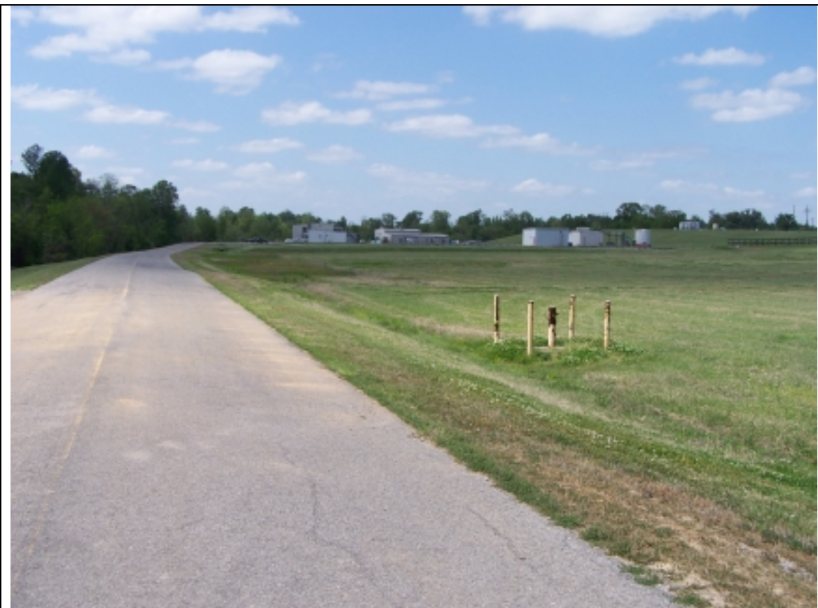
Photograph 11 – South Levee Road, Brooklawn OU, West 4/6/10
